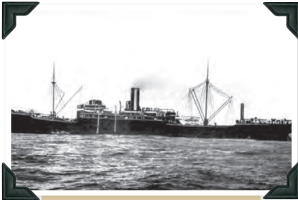
ABOVE: The SMS Wolf was a converted freighter fitted with six 15-centimetre guns, multiple smaller guns, four torpedo tubes and more than 450 mines.
